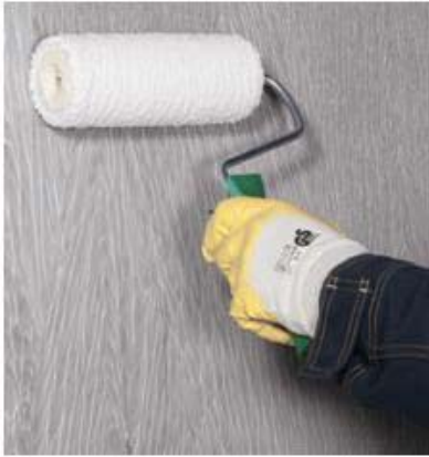
Application of MC-DUR 111D
